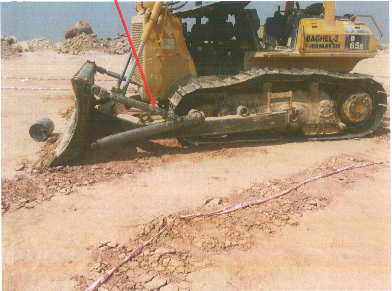
Photo 7 Position of deceased immediately prior to incident. Deceased was lying under the machine draining oil from sump and passing to fellow employee sitting on left track . Position of deceased lying under machine prior to incident
