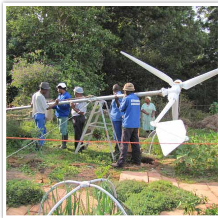
Community members raise a 1KWh turbine in Claridge, KwaZulu-Natal, South Africa. Photo credit: Jane Harley.
