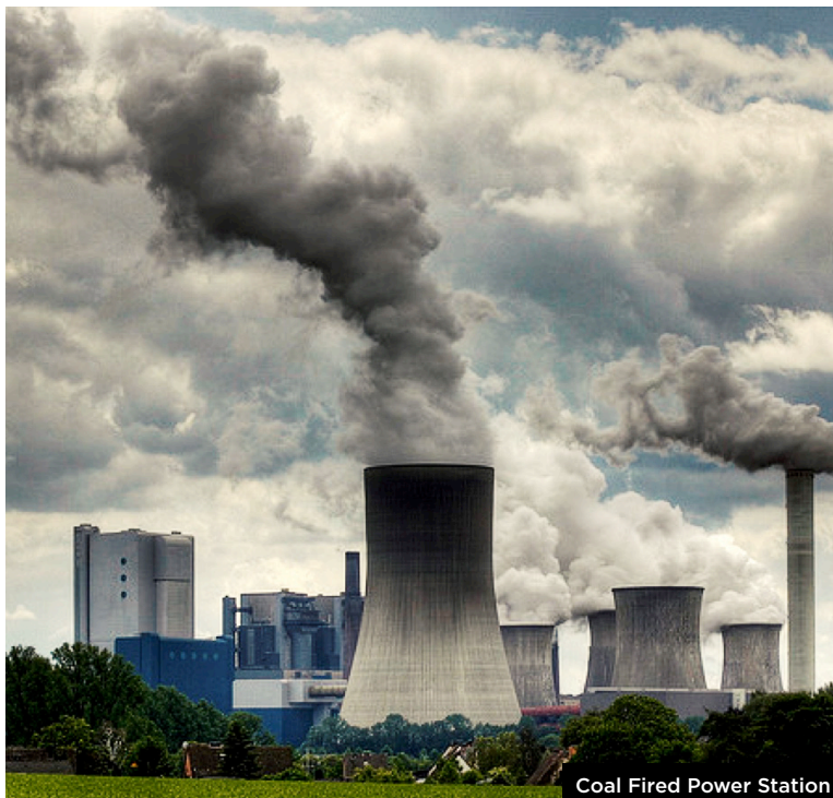
Coal Fired Power Station
