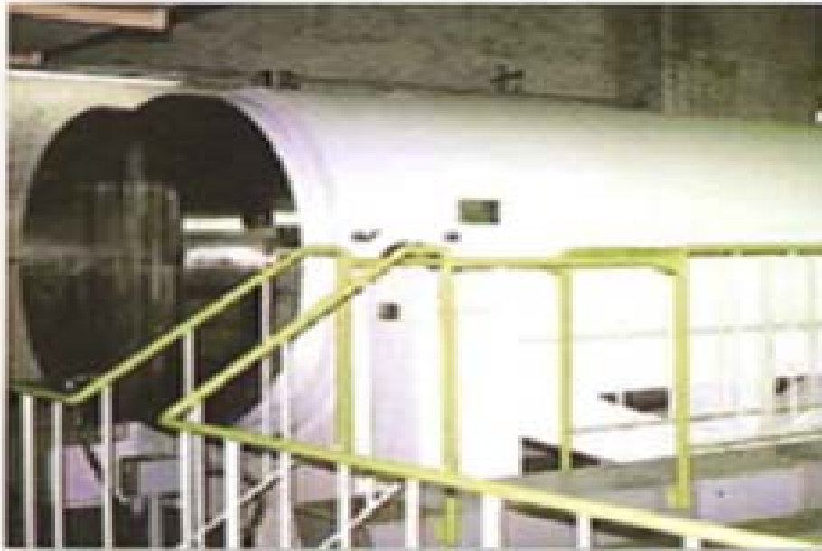
Spent Fuel Storage Cask at the Dai-Ichi Site
