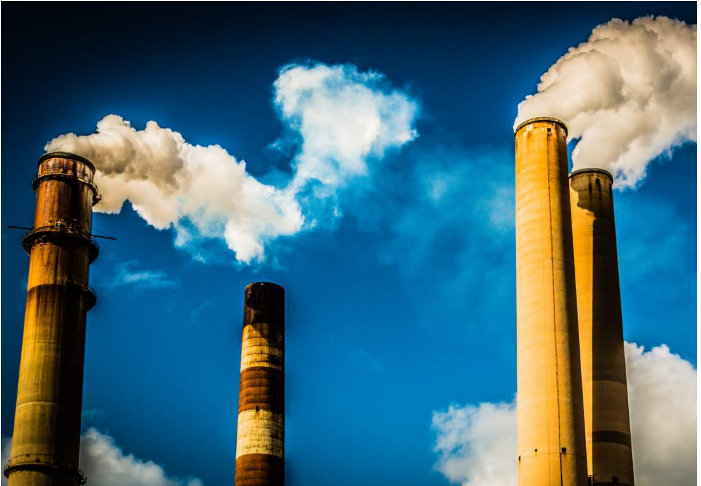
ABOVE: Smoke stacks at Teco Big Bend Station, Florida, 2013. Credit: Bjorn Christian Finbraten, Flickr, Creative Commons.
