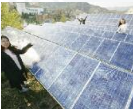
15 kW of solar power installed on the roof of KFEM office has been operated since 2001, known as the first solar plant in Seoul. © KFEM
